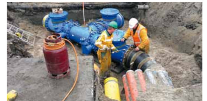
Reconstruction of the underground infrastructure at the Drachtsterplein square.
