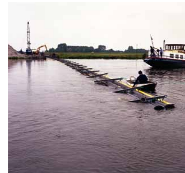
Construction of a combined submersed pipeline, carried out by the Hattem location.
