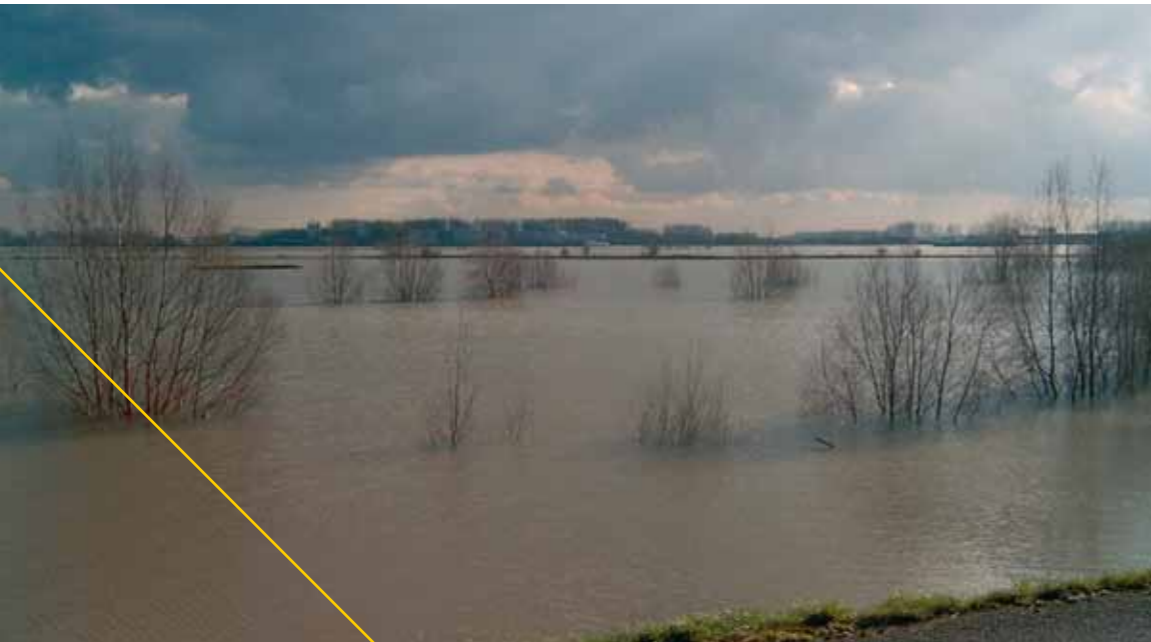
The Waal Dike near Ochten almost breached.
