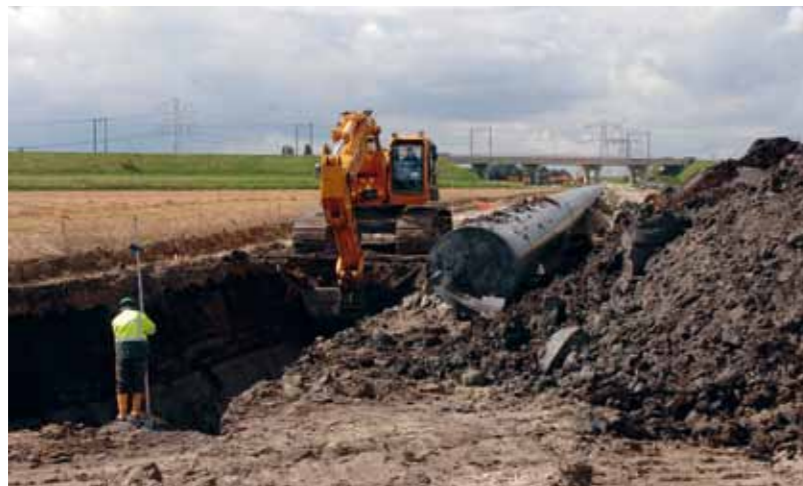
Construction of a 55 kilometre 48" gas pipeline for Delta Energy.
