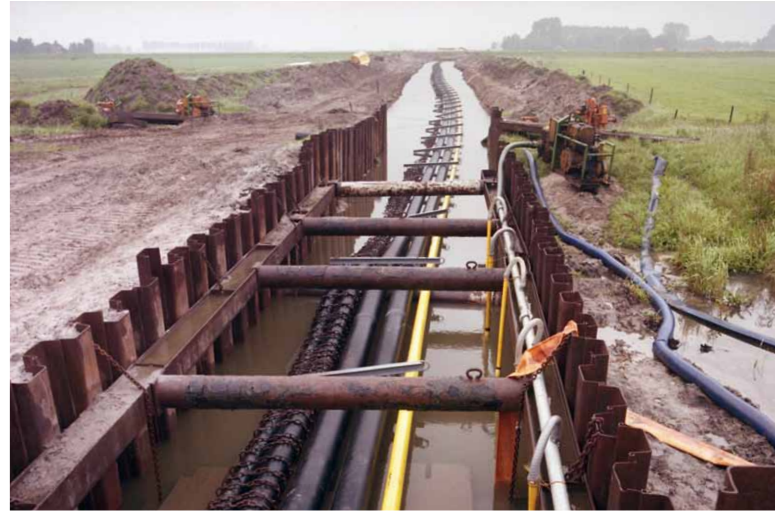
Construction of a combined submersed pipeline, carried out by the Hattem location.
