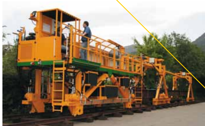
The pipeline is transported through and installed in a tunnel with a custom train that was built especially for this project.
