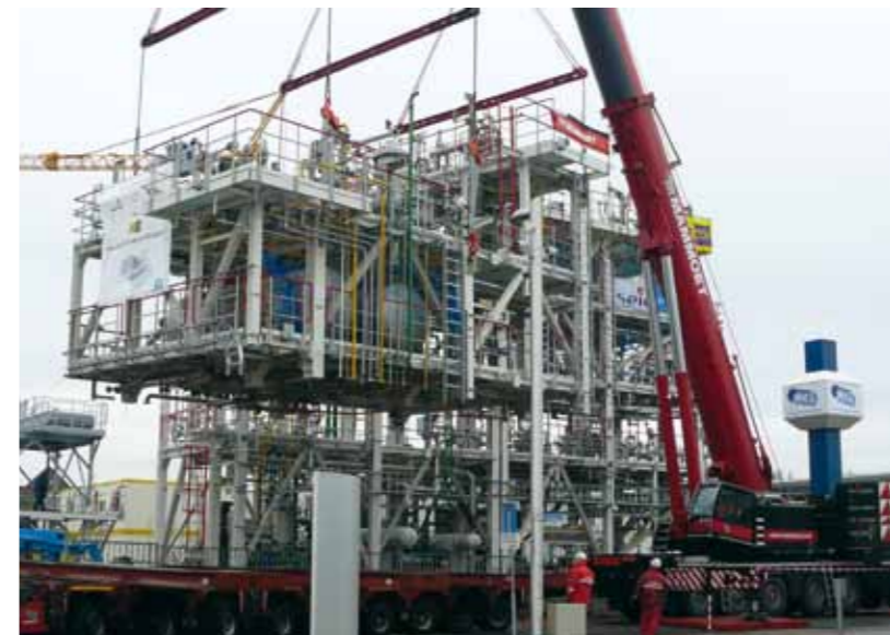
MCL constructs a 250 ton CO 2 capture system.
