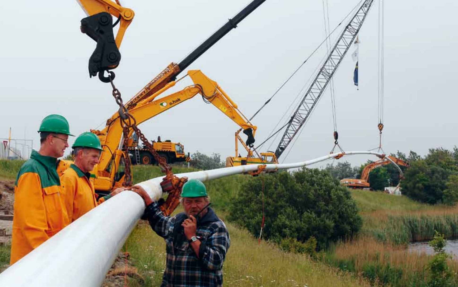
A special, two-sided 1,300 meter drilling, right through the Lauwersmeer nature reserve.
